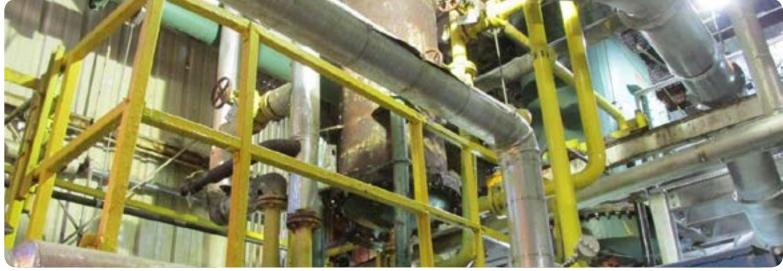
The 29"-diameter steel vessel had been previously patched two times with a "non-code repair", and needed a stronger, the code compliant repair. Steel thinning had resulted in the vessel's inability to withstand normal operating pressures. HJ3's CarbonSeal system was installed in 2 days and returned the vessel to its original strength, without requiring a shutdown.
