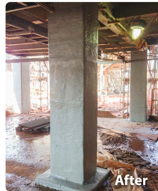
Some of the completed columns with topcoat to prevent chemical degradation
